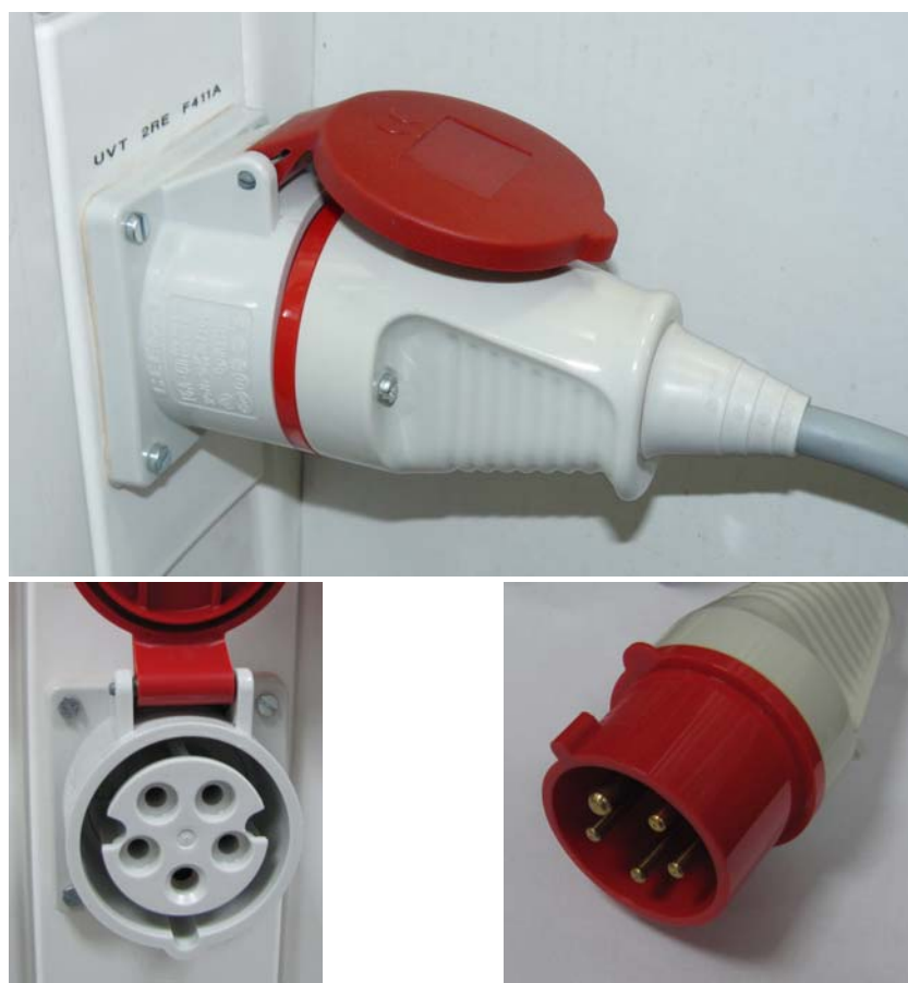
Figure 4-2. Wall mounting of receptacle and plug of mains power cable
