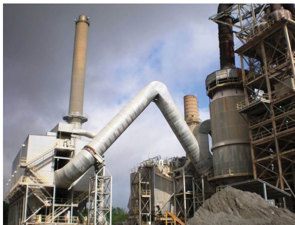
Figure 3: View of the Midwestern cement kiln
